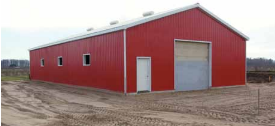
Preparing for 2010, the Pais family has built a red-sided, 40 by 80 foot barn. They put up the structure themselves and have plans to add a cooler unit. Photo by Hugh McElhone
