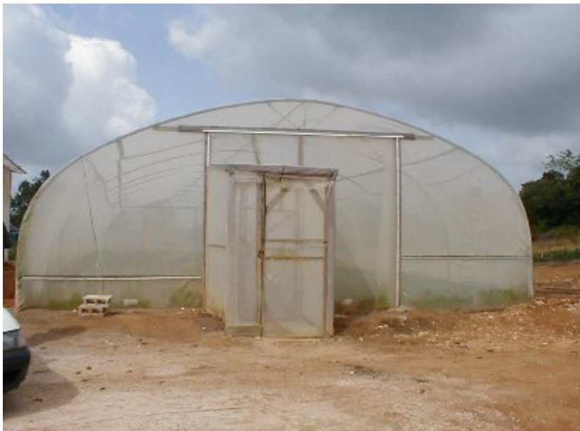
Existing high tunnel at Devon property currently used for sweet potato planting material. This design is more wind resistant; however it does not provide ideal growing temperature. The project will investigate the potential for using the best design features of both to come up with a wind resistant, cooler high tunnel that will be affordable to small farmers.
